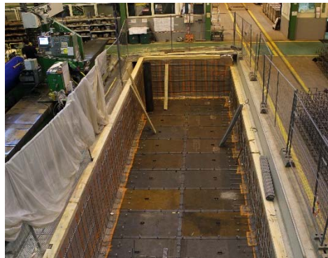
Figure 9: Welded steel plates for shutting
