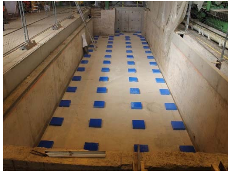
Figure 8: Discrete elastomer pads in the foundation-pit
