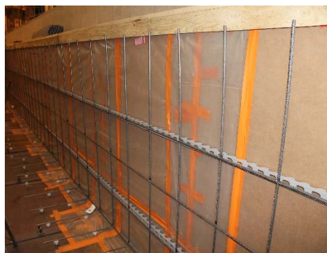
Figure 10: cardboard lateral gap
